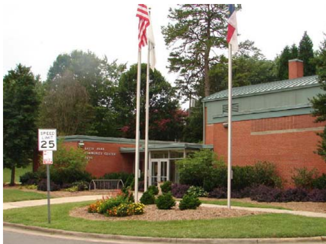
Charlotte Bridge Center 510 Park Ave, Charlotte, NC
